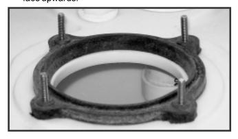
Place toilet on studs and secure with four washers and four nuts.
