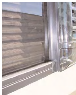
Cut Wiper Gasket FIG T
