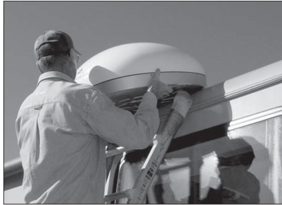
Figure 5: Carrying the Antenna to the Roof
